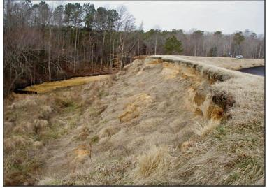
Figure 8—Slumping on the downstream face of a dam.
