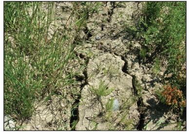
Figure 20—Transverse cracks can be an indication of dam instability.
