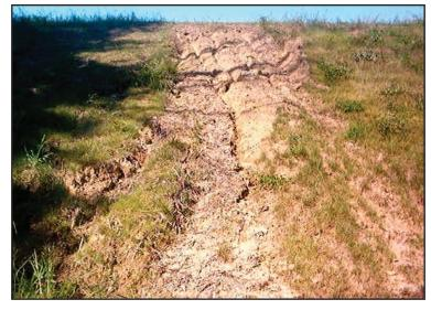
Figure 12—Erosion on the downstream face of a dam.
