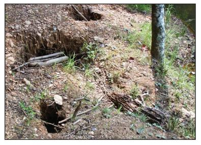
Figure 16—Rodent holes in the dam face can cause dam failure.
