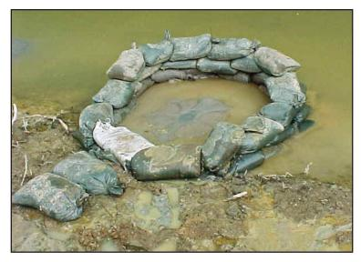
Figure 28— Sandbags surrounding a boil on the downstream side of the dam.
