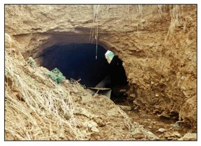
Figure 32—Piping of water alongside an outlet pipe.
