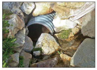
Figure 34—Rock failure around an outlet pipe.
