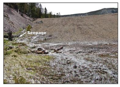
Figure 30—Seepage at the abutment contact (groin) can lead to dam failure.
