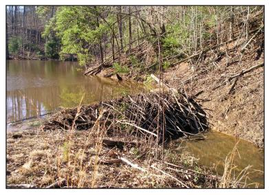
Figure 38—A blocked spillway channel may cause overtopping of the dam.
