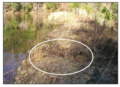
Figure 24—Low areas in the crest of a dam reduce the freeboard.
