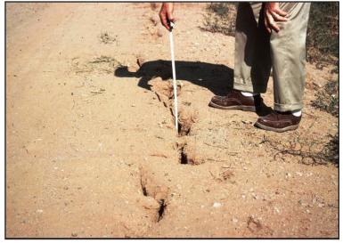
Figure 22—Longitudinal cracks can be an indication of dam instability.
