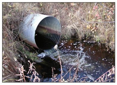
Figure 36—A scour hole at an outlet erodes the toe of the slope.
