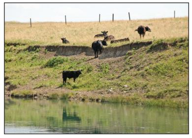
Figure 18—Livestock paths on dam faces can lead to dam erosion.
